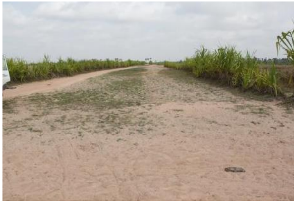
Canal before rehabilitation at CODEC, Kampong Thom province
